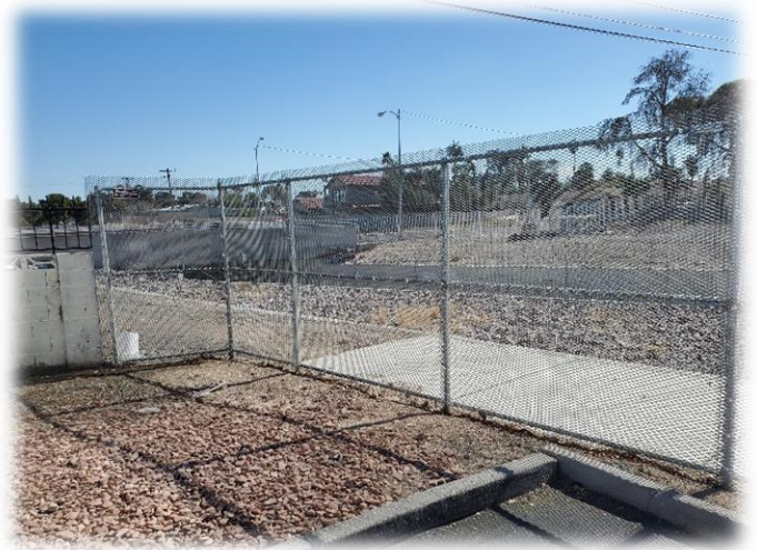
Exclusionary fencing along Flamingo Wash. (Photo by CCRFCD).
