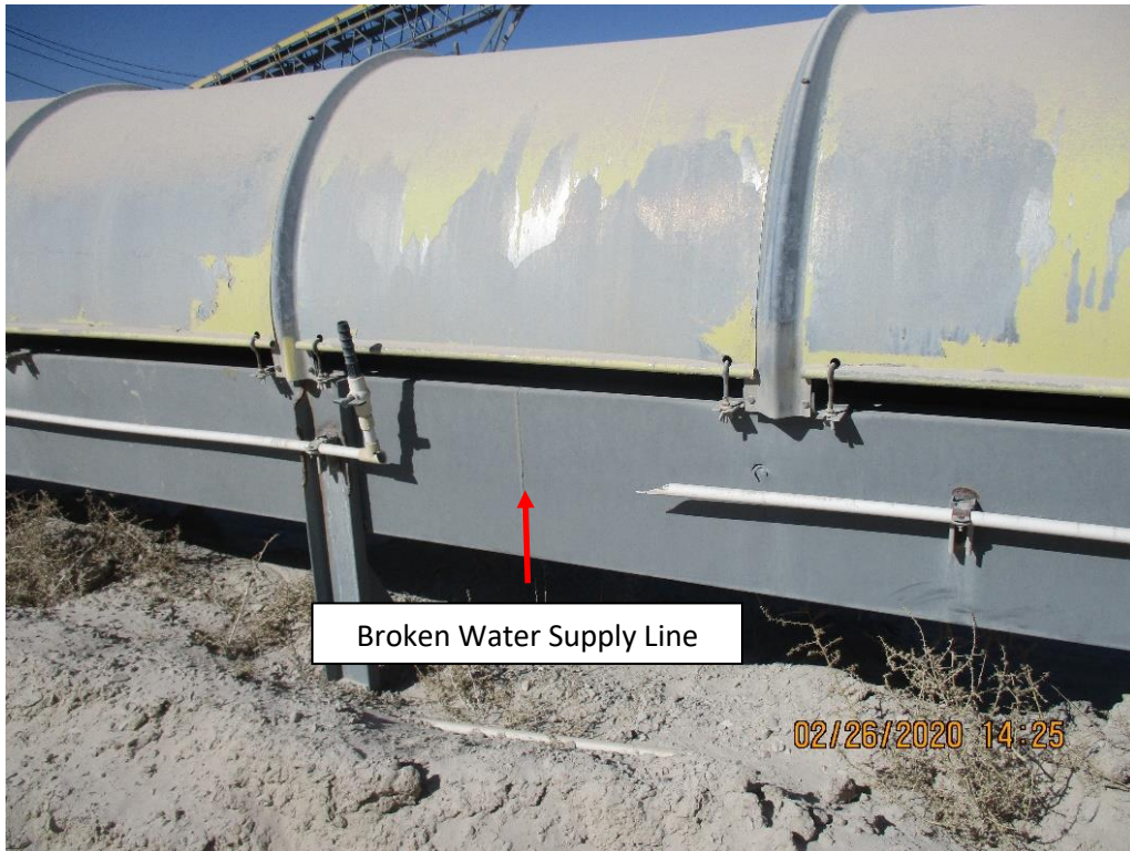
Photo 4 – Another Example of Water Sprays Not Operating
