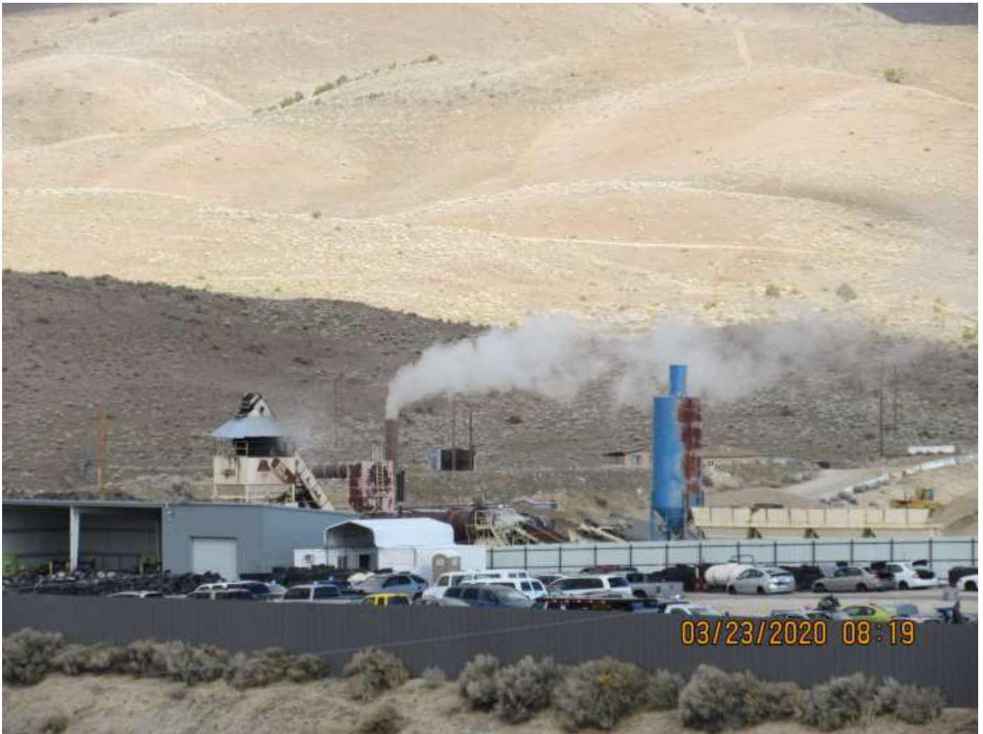
Photo 2- System 02 (S2.001) Emitting High Opacity Smoke
