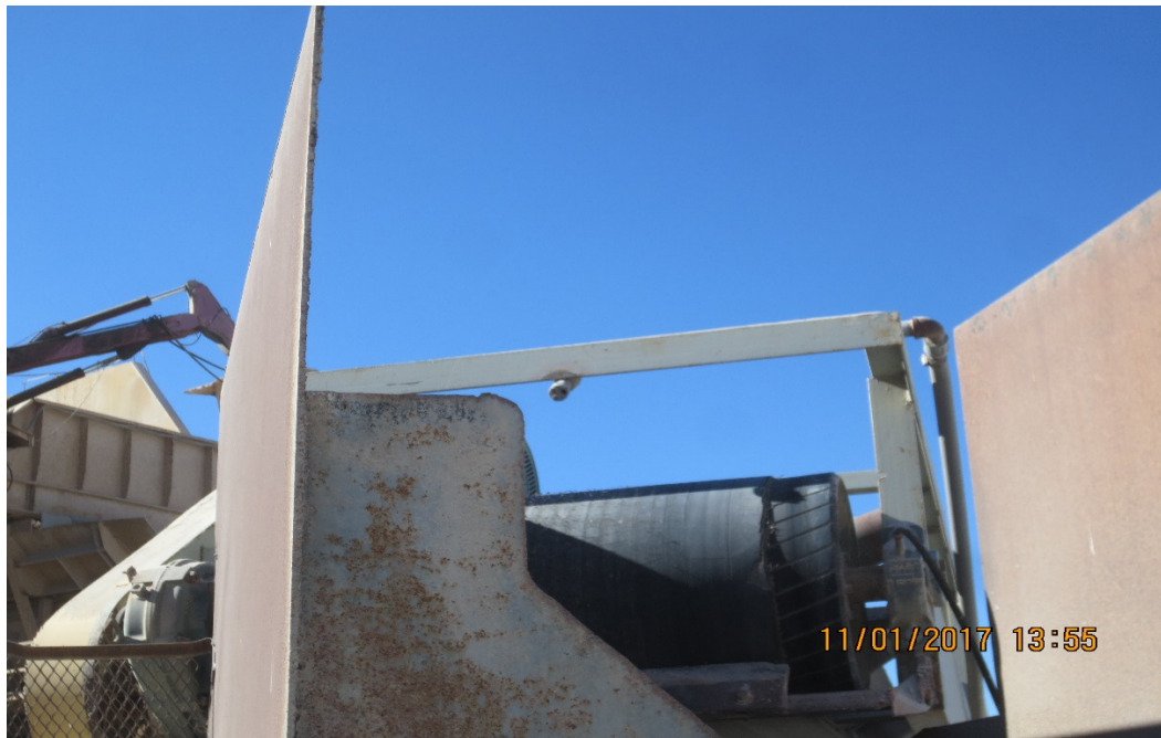
Photo 2: Water spray not in operation.
