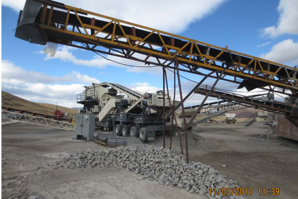
Photo 1: Unpermitted portable crushing and screening circuit.
