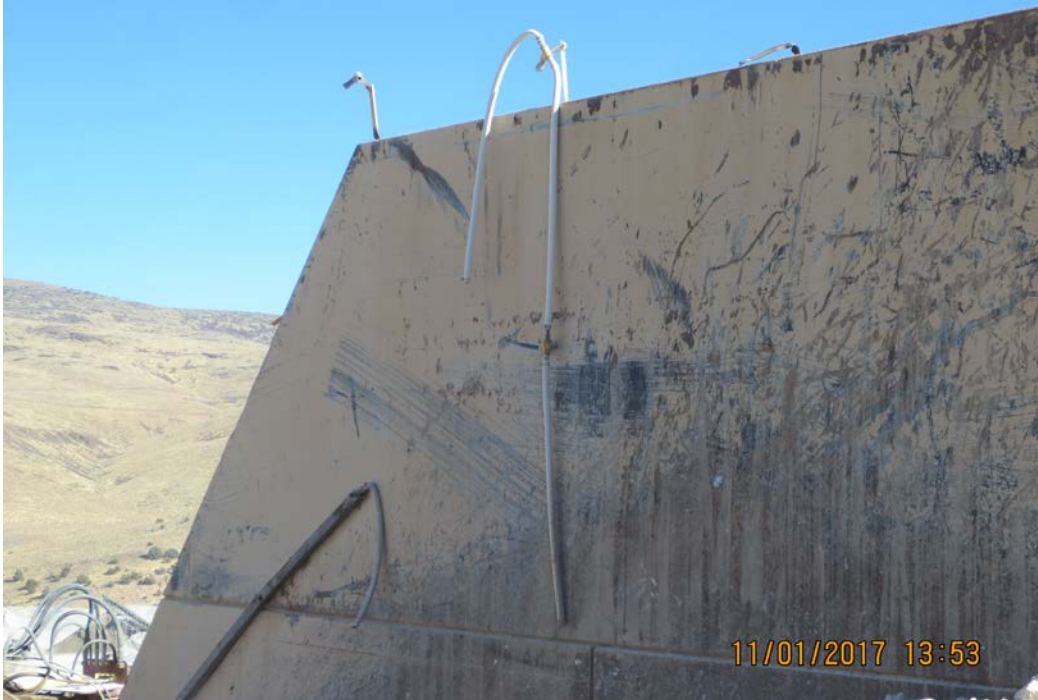
Photo 1: Damaged water lines for the pneumatic fogging water sprays for System 1.
