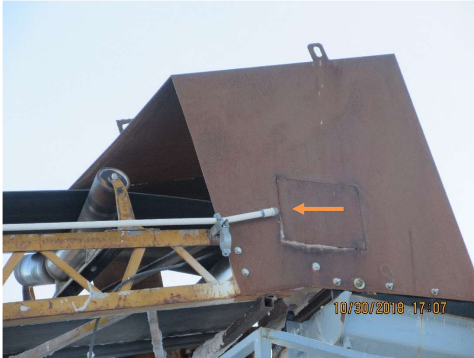
Photo 1 - Water Supply Line for Waters Sprays Capped Off
