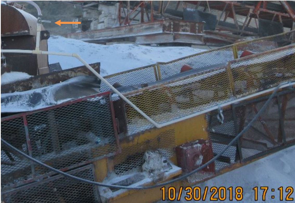
Photo 3 - Valve Closed for Water Supply Line for Water Sprays
