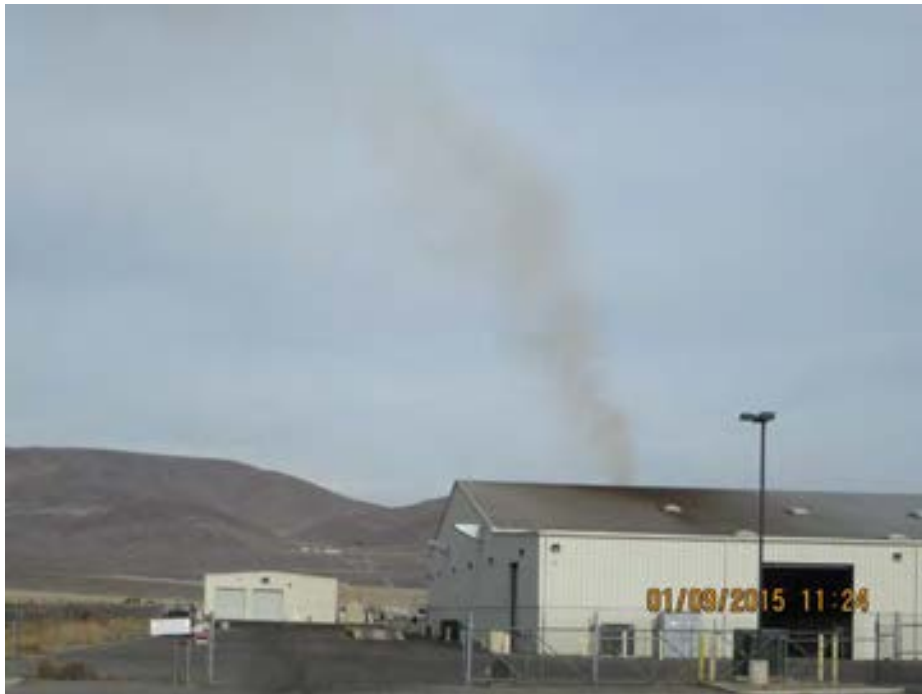
Photo 4: Photo taken during BAPC visible emission observation showing average opacity of 31.25%. Evidence of historical stack emissions shown by discoloration on roof of building.
