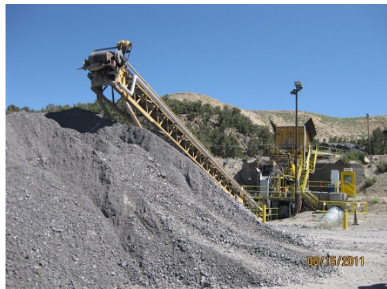
Systems 1-5 – Ore crushing and screening systems.
