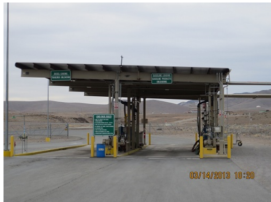
System 2A - Facility Fuel Loading Rack System
