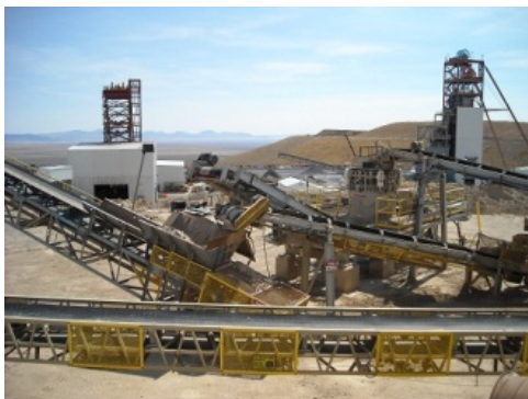
Ore crushing and screening systems.
