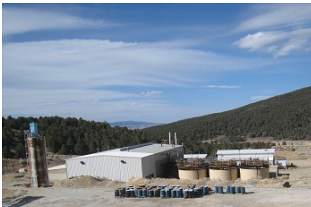
System 6 – Refinery Equipment in building to left of (yellow) carbon-in-leach tanks.
