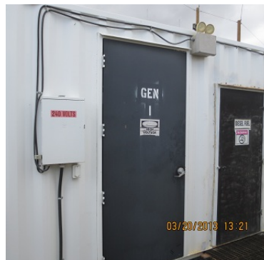
System 52: (2) Substation Emergency Gensets (2,836 HP each).
