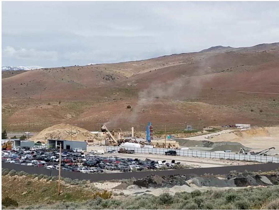
Photo 1: Visible emission observation showing average opacity of 22.5% on April 25, 2017.
