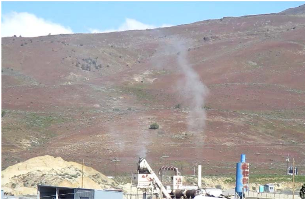
Photo 2: Visible emission observation showing average opacity of 28.5% on April 28, 2017 (image taken from BAPC video).
