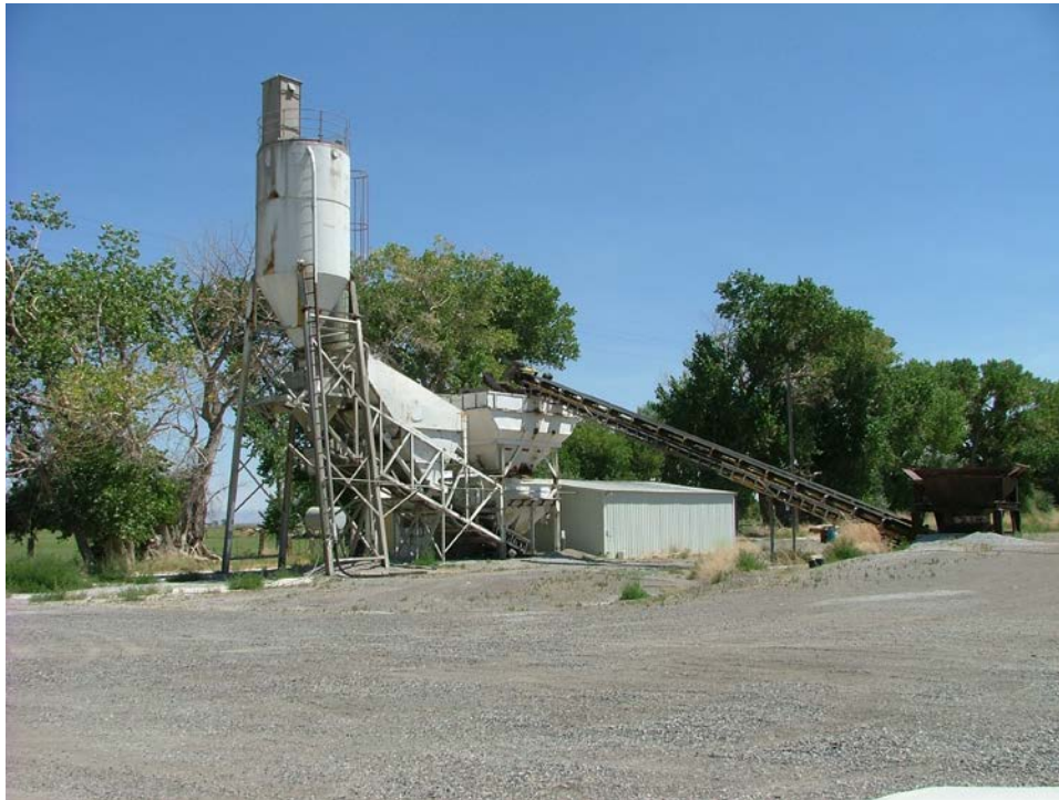
Photo 1: L. Mackedon & Sons, Inc. Concrete Batch Plant.
