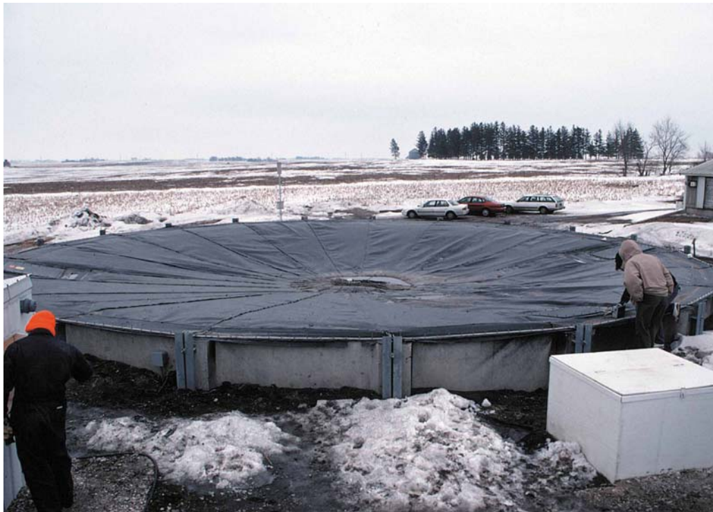
Figure 7.6. Covered manure tank generating methane in Iowa.
